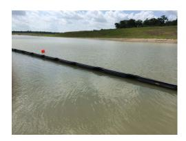
ABASCO medium duty diversion baffles are ideal for controlling flow and circulation in wastewater treating ponds, to eliminate dead zones, increase detention time, and improve treatment efficiency. Heavy duty tension members at the top and bottom of the curtain and UV/chemical/acid/base resistant 30 oz. Elvaloy coated fabric with additional skirt fabric options. Custom designs upon request based upon application requirements.
